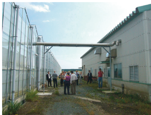
Toyota Floritech transferring heat and CO2 to greenhouse
